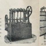
POMPA DI PRESSIONE PER PRESSE IDRAULICHE.
